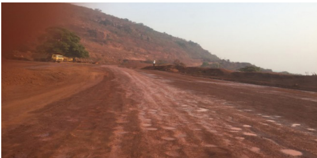
Figure 3. Conventional water sprinkling resulting in muddy haul roads.
